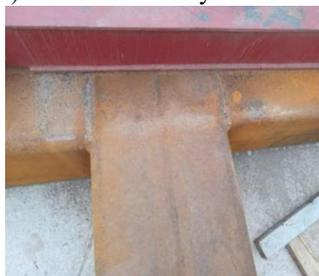
**Figure 8** Steel Platform Welding
