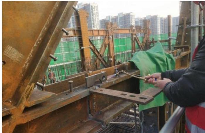
**Figure 2** Welding Preheating Treatment
